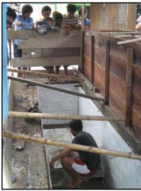
built into the ground and the other tank built above ground. A pump drew water from the ocean to flush the upper tank and excess water accumulating in the upper tank was sent by gravity feed into the lower tank to flush that system. Water from the bottom of the lower tank was pumped up to ground level where it was purged from the system into a
