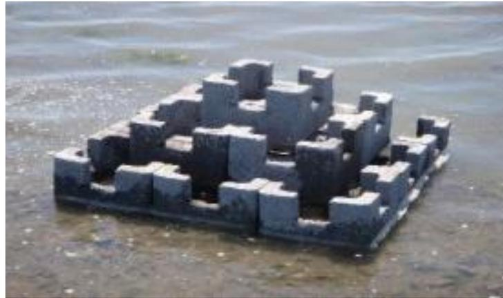
**Figure 3** An example of an oyster castle used in experimental and small-scale restoration projects since 2007 (Allied Concrete 2011).
