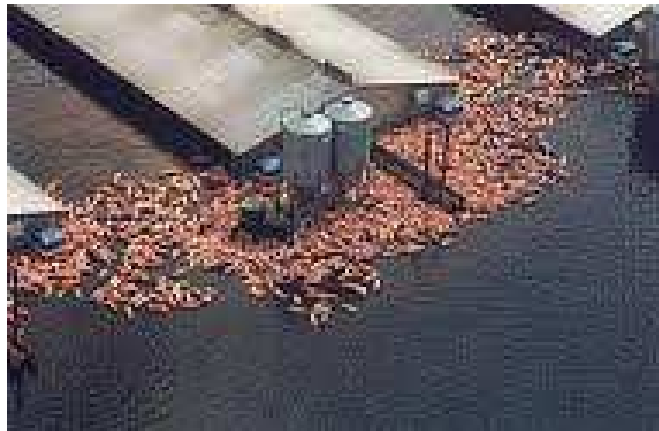
Figure 8: North Carolina Hog CAFO after a Hurricane Floyd 1999. Estimates of hog deaths in this flood ranged widely from 30,050(officially reported)-400,000 110
