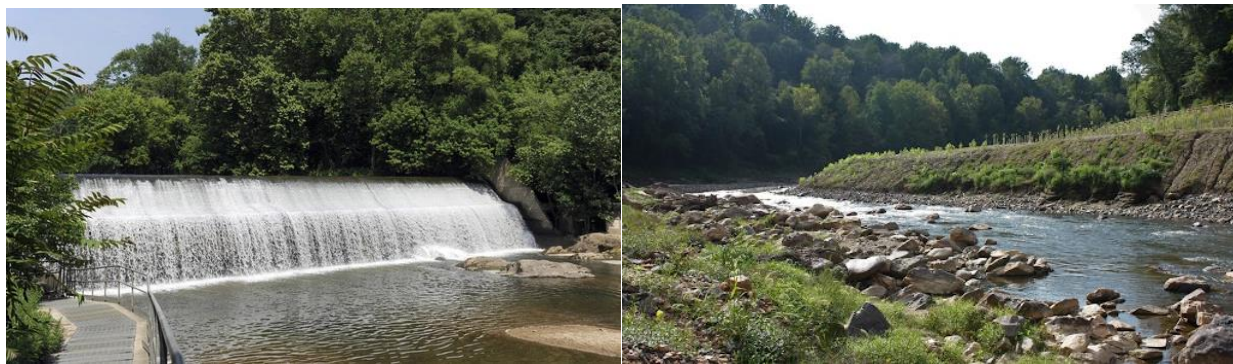
Figure 2. Bloede Dam before removal in 2018 (left) and the former dam site after breaching and full bank and streambed restoration (right). Images from Maryland Department of Natural Resources.
