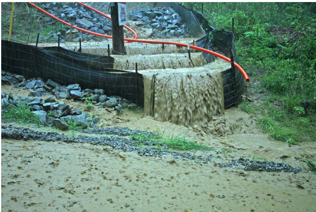
Figure1: A photograph of the failure of the net system in July 17 th , 2007, Asheville. The rainfall event inducing this sediment erosion was usual for this summer period. Note the sequence of nets and the large sediment erosion passing through the nets. Currently, this kind of protection meets the state ordinance.
