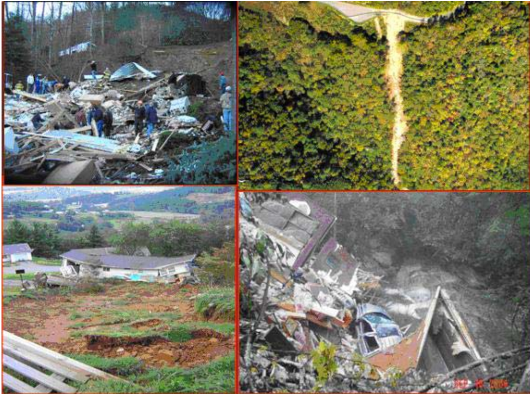
Figure 8: Landslide hazardous Photo Top Left: Maggie Valley home destroyed by embankment failure, December 13, 2003. One occupant of the destroyed home was killed. Photo Top Right: Embankment failure-debris flow along the Blue Ridge Parkway triggered by rainfall from Hurricane Frances, Sept. 6-8, 2004. Photo Center: Home destroyed by embankment failure-debris flow near Jonas Ridge, Burke County during Hurricane Frances in 2004. Photo Bottom Left: Home destroyed by an embankment failure-debris flow in the White Laurel community during Hurricane Frances. 7
