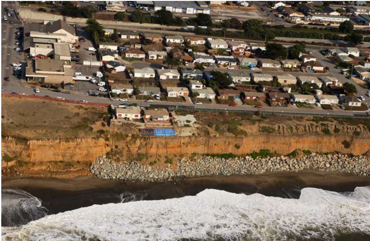
Plate 1 Pagan OTD, hazardous cliff and reinforcement visible
