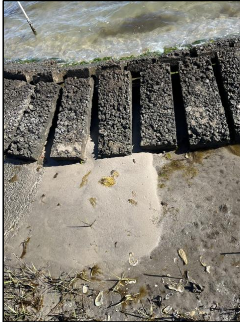
Figure 2. Living shoreline with sill made of QuickReef . Sediment accretion is visible landward and oyster recruitment waterward. 3
