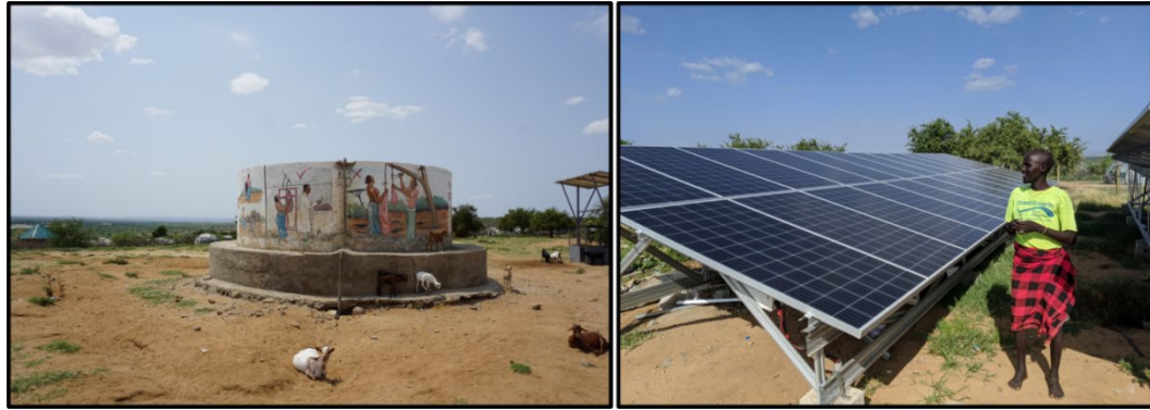
Figure 29: Examples of market infrastructure in Illeret. Left: Water cistern with solar pump located in the Kerech community. Right: Solar array installed in December 2019 and turned on in January 2020 through a partnership between Kenya Power and German energy company, GIZ. This array provides moderate power to small businesses, households, and community buildings that are constructed in a permanent fashion. Expansions to the solar grid planned in the near future.
