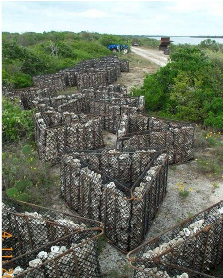
*Figure 4 Mad Island interlockable Reefblocks™ ready for placement (picture courtesy of Coastal Environments Inc (Randy Sunde)*
