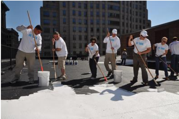
Figure 32. NYC Cool Roof Volunteers. Source: http://www.coolroofs.org/newsletters/CRRC_Summer_2010.html
