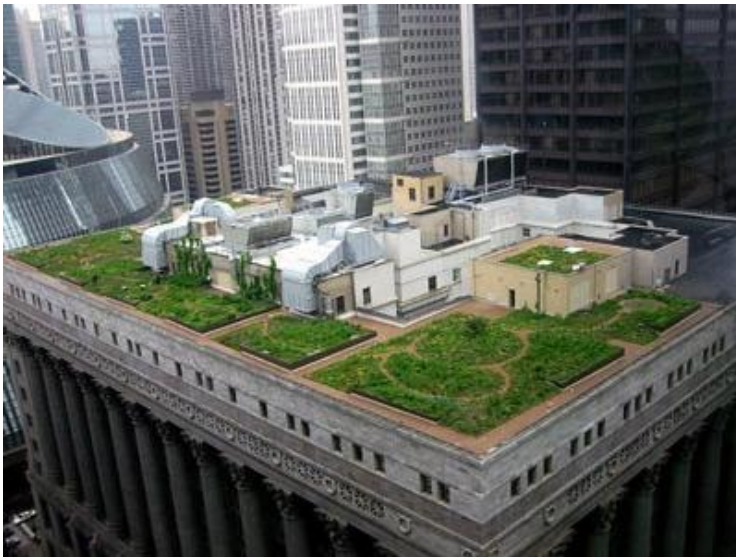
Figure 31. The Chicago City Hall green roof.
