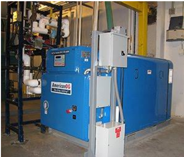
Figure 24. Cogeneration System. Source: http://www.cleantechny.blogspot.com/
