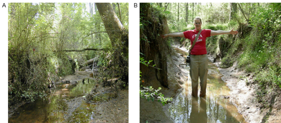
Fig. 2. (A) A photograph of Sandy Creek at WT-1 within the SWAMP project site taken on 19 May 2005, prior to construction of the new stream channel, illustrates the rectangular channel profile and the large degree of channel incision that had developed throughout much of the project area. For reference, the left bank of the stream in this photo (flow is toward the reader) is approximately 2.5 m. (B) A heavily incised tributary of Sandy Creek in the SWAMP site upstream from WT-3 (see Fig. 4 for Water Transect (WT) locations site locations).
