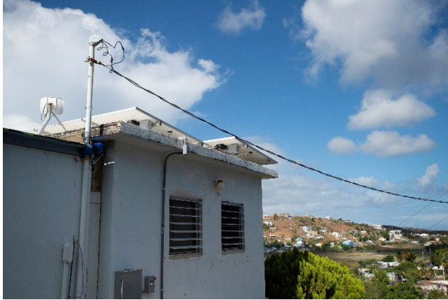
Problems with feeder equipment in some neighborhoods caused connection delays and operational issues. Photo courtesy of EDF.
