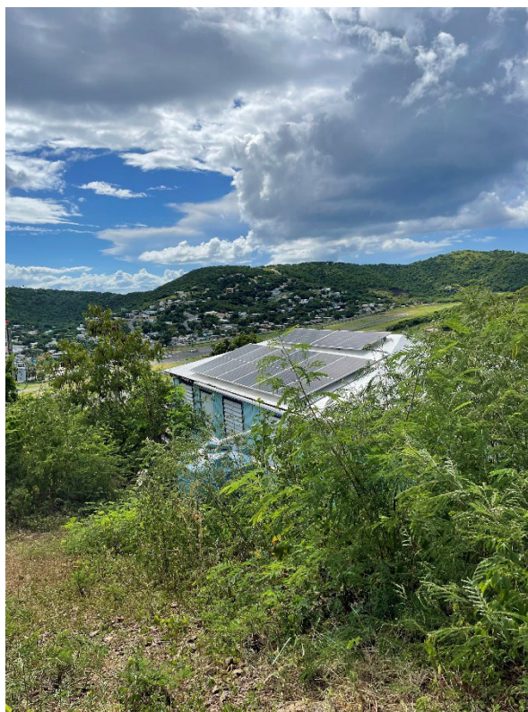
A solar-powered house in Culebra. Photo by Jenny Mandel.
