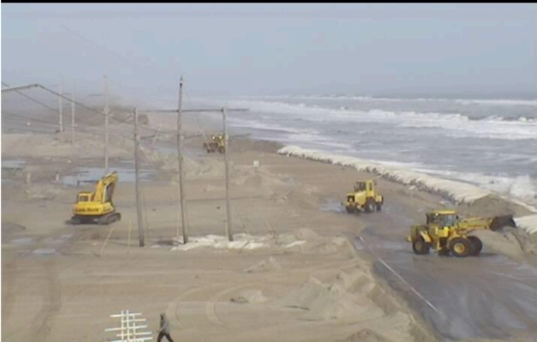
Figure 3. NCDOT clearing sand from NC 12 north of Rodanthe, NC on March 11, 2013 (NCDOT, 2013a).
