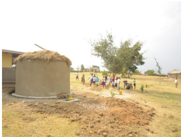
Figure 1: IRWH tank at a primary school
