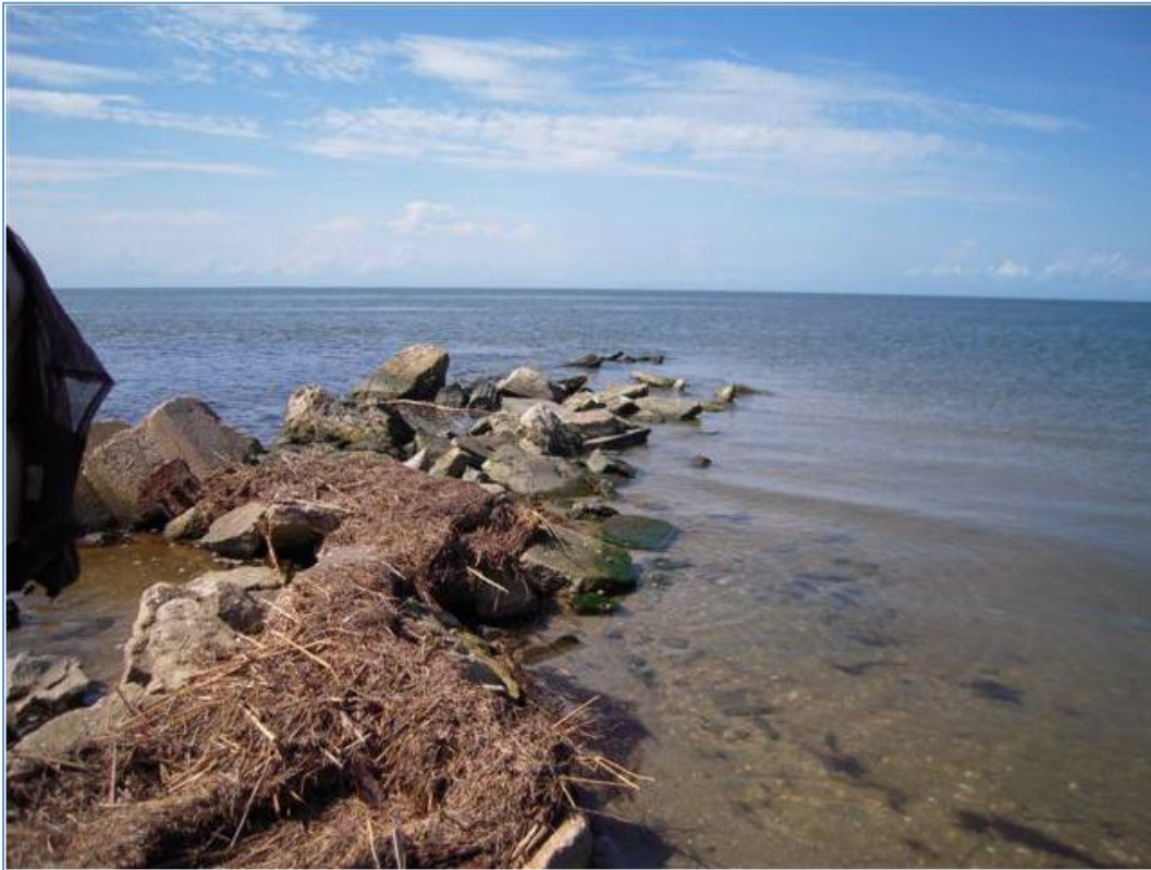
Figure 3 - Existing Jetty between Old Slough and Pamlico Sound Shoreline
