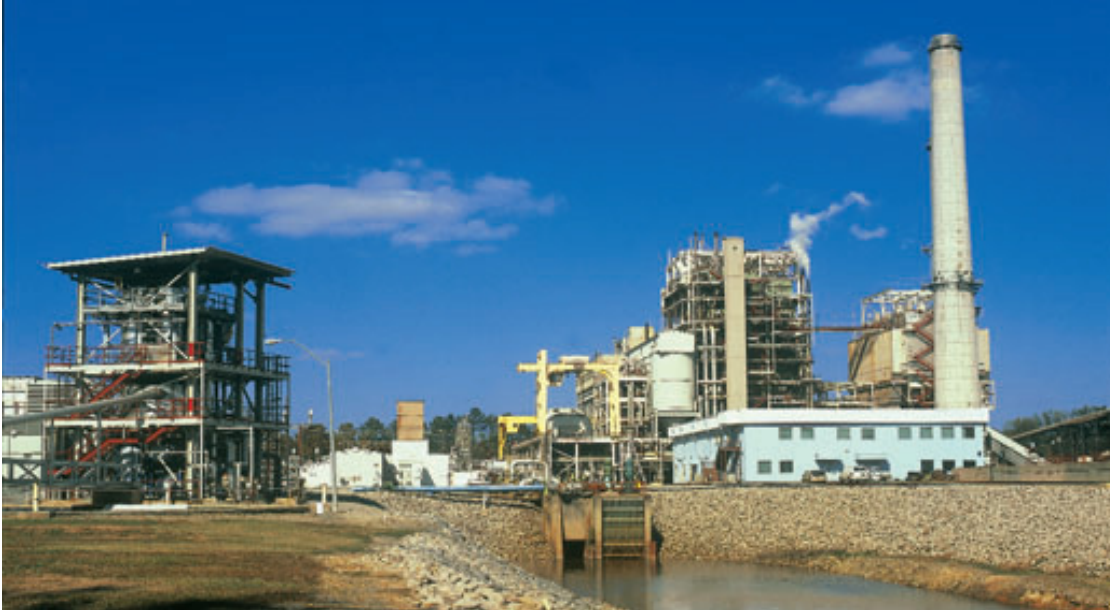
Progress Energy's Lee Plant is located on the Neuse River near Goldsboro N.C.
