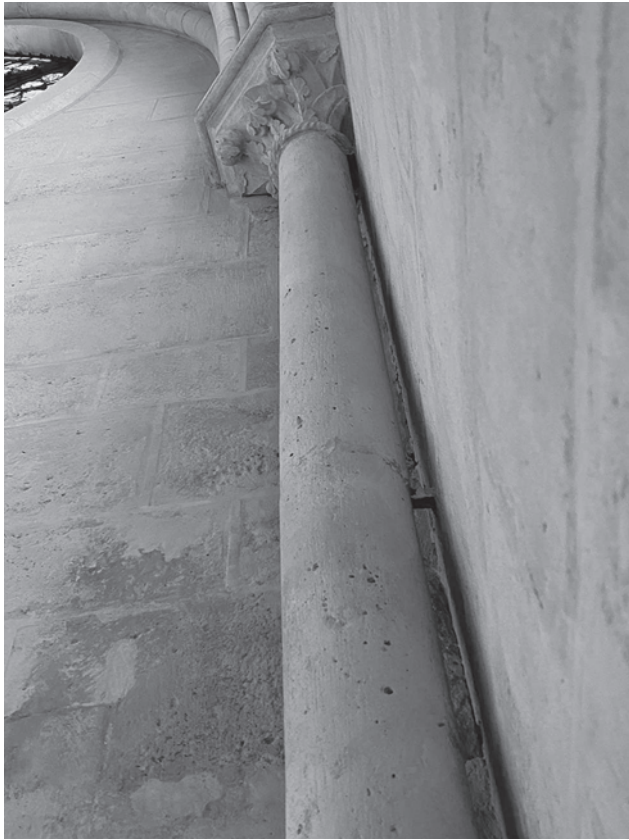
Figure 10 Notre-Dame in Paris, detached shaft in the southeast corner of the south transept arm (author's photo).
