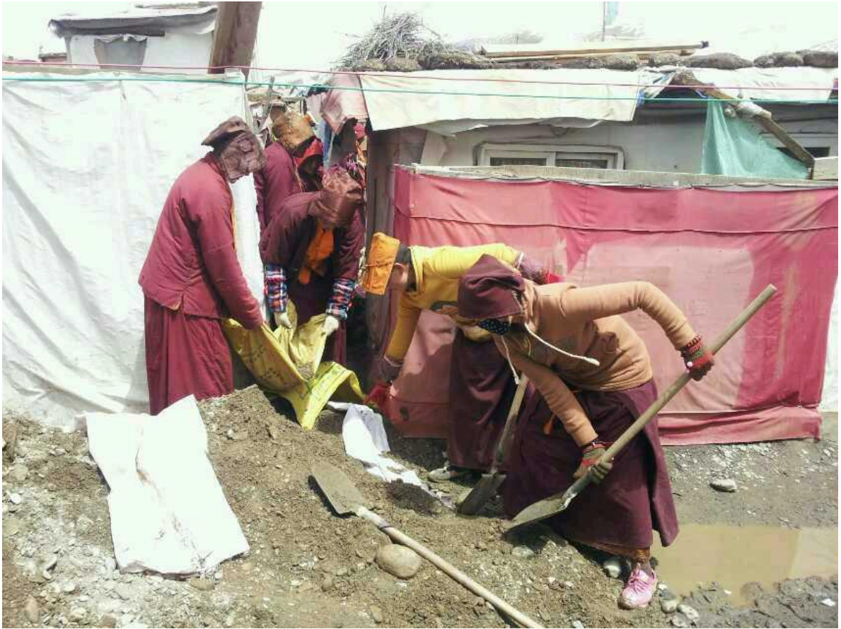
Figure 7: Nuns are building a hut. Photo by Yasmin Cho (2013).
