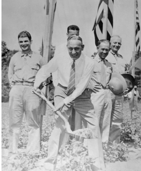
Figure 18: Mayor Lucien P. Burns breaking ground at Craig Air Force Base. Courtesy of Old Depot Museum.
