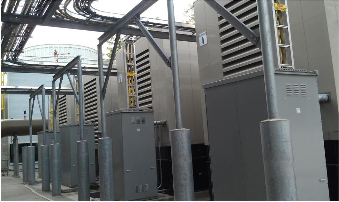
Figure 1: Diesel-powered Emergency Generators at Duke Chilled Plant #2
