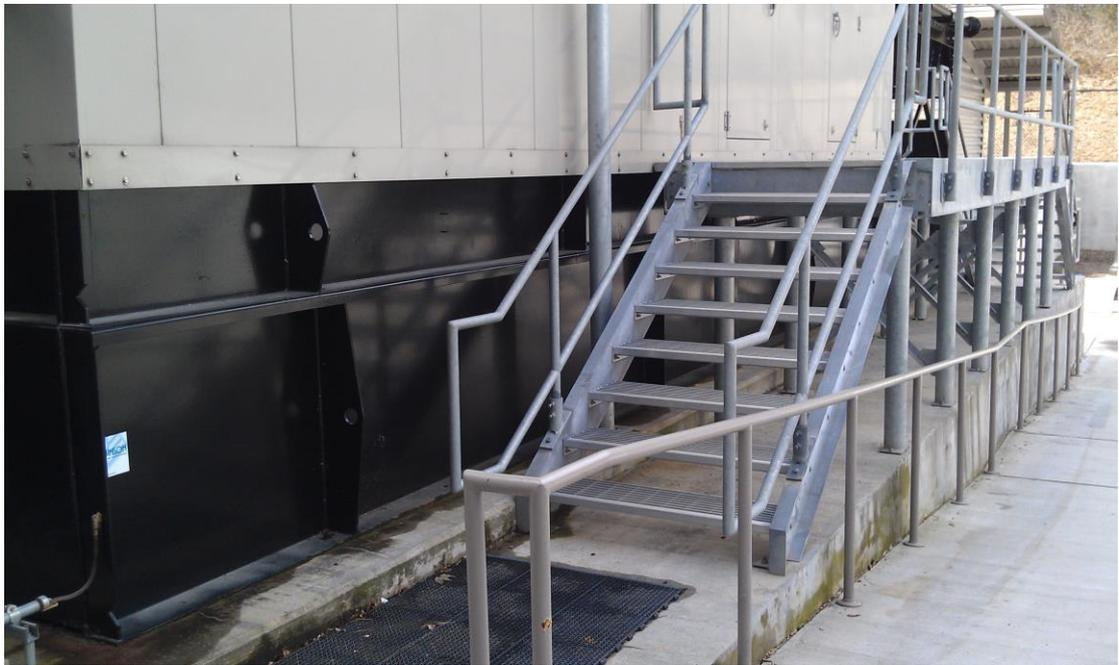
Figure 2: Diesel Fuel Tanks below the Generators
