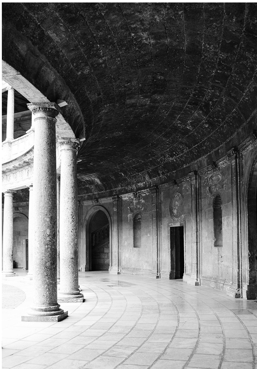
FIG. 1 – Pedro and Luis Machuca, annular stereotomic vault, 1562-1569, courtyard, Palace of Charles V, Granada. Photo © Sara Galletti.
