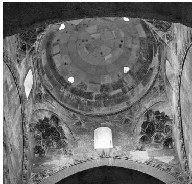
FIG. 8 – Dome with single, helical course, Caravanserai of Sultan Han, Sultanhanı (Aksaray), 13 th cent. © Claude Valette (Own work) [GFDL, https://commons.wikimedia.org/w/index.php?curid=15015965 ].
