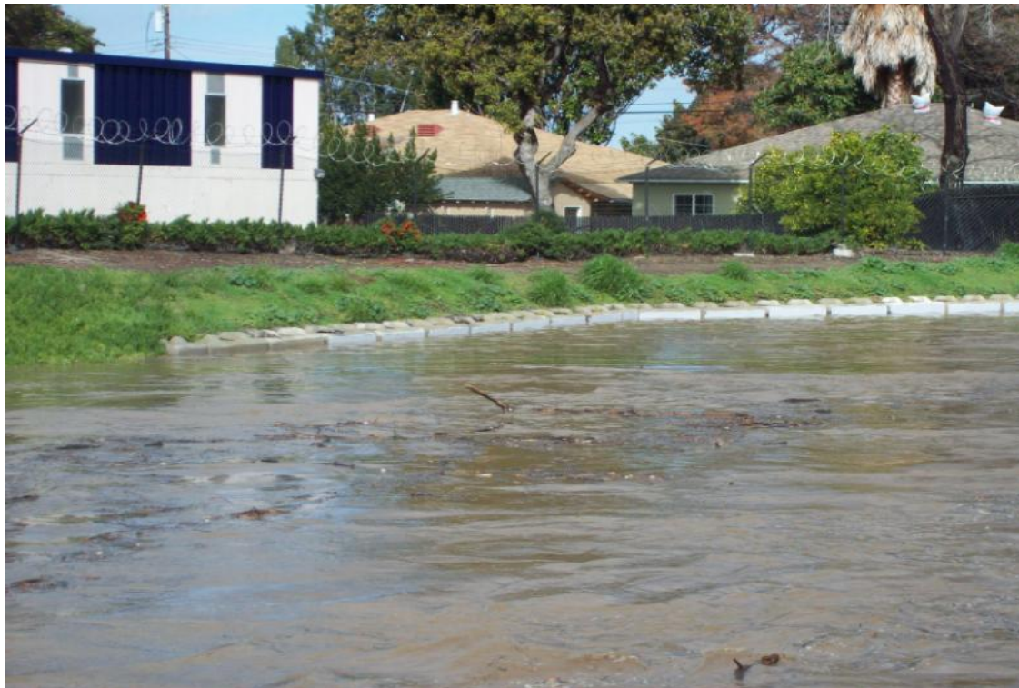
Figure 8: San Francisquito Creek near maximum capacity adjacent to homes in the Gardens Source: City of East Palo Alto, 2010
