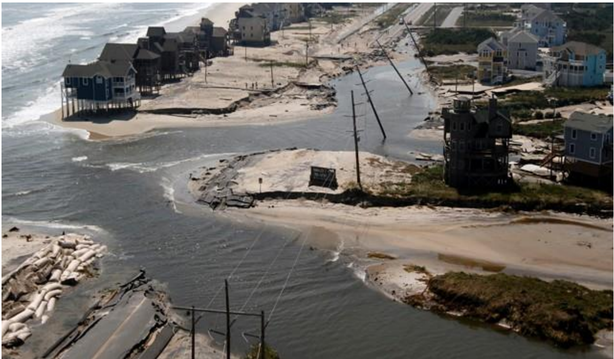
Figure 9. One of two breaches of NC 12 after Hurricane Irene in 2011 north of Rodanthe, NC (Associated Press, 2012).
