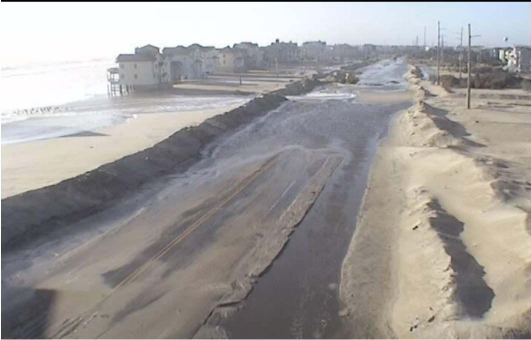
Figure 2. Sand and water on NC 12 north of Rodanthe, NC on March 9, 2013 (NCDOT, 2013a)
