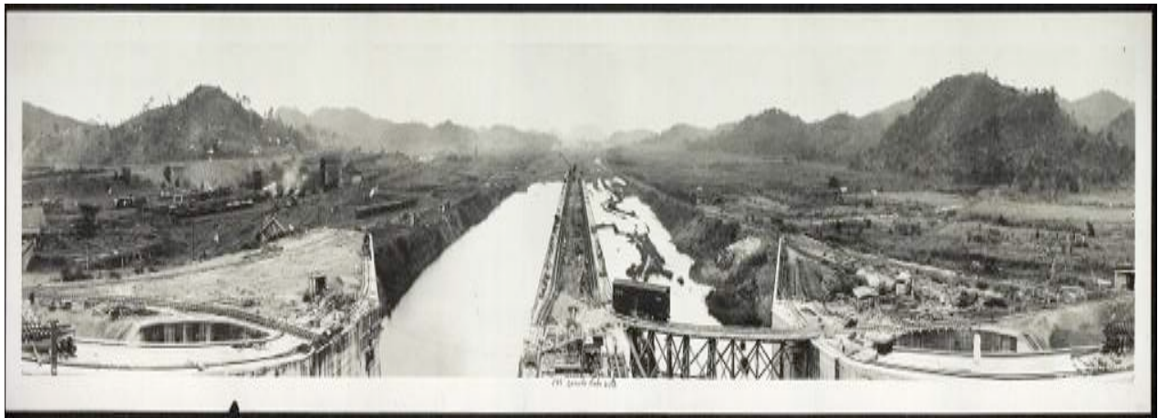
National Archives: Panoramic photo of construction of Miraflores Locks in 1913. Cocoli is behind hill to the left.
