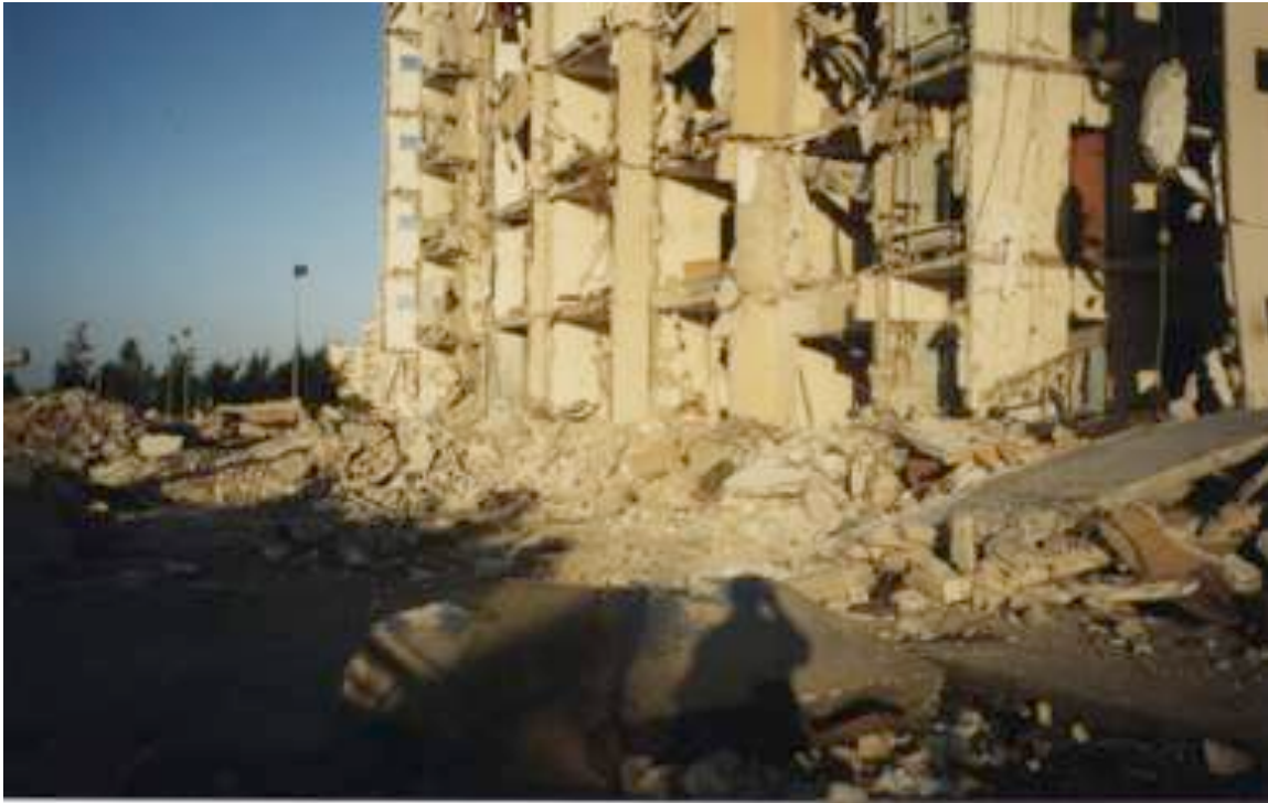
Khobar Towers Building 131. Photo taken a few days after the blast.
