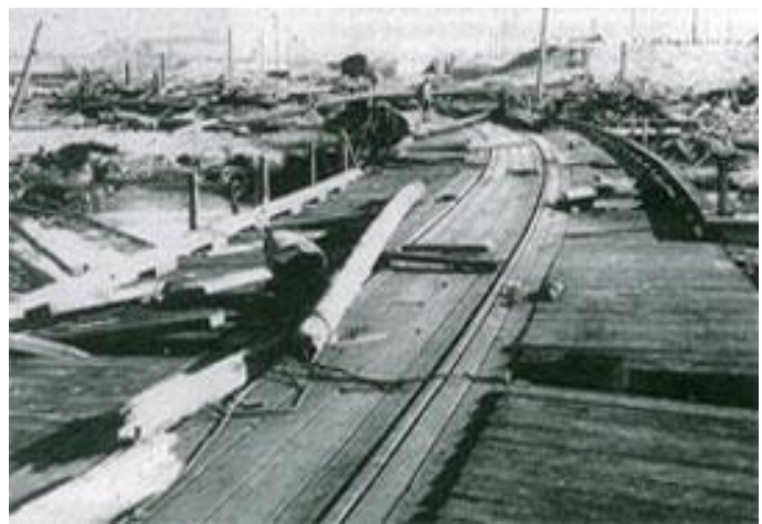
Figure 9 - Images of Explosion at Port Chicago (NPS, 2012)
