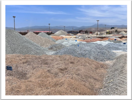
Figure 3 Ore Stockpile in Veta Dorada's Processing Plant
