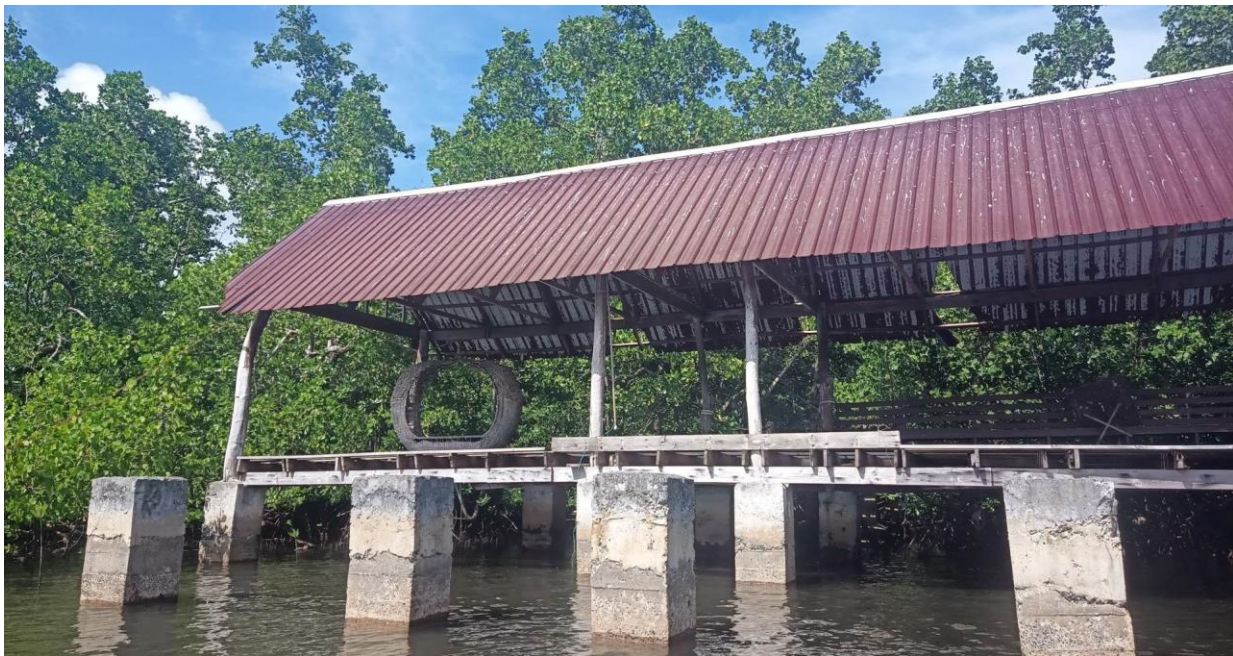
Figure 4 Papago resort boathouse, located at the eastern terminus of the boardwalk from the resort. There are 6 concrete piers in total, all of which measured at least one 2.2m lidar point and an average of 2.18m
