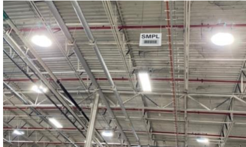
Appendix 2. Solar Tubes in the Warehouse
