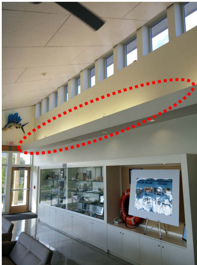
Figure 14. The Repass Center common area has lighting fixtures hidden behind recessed areas that render visual assessments difficult. Floor plans and other information were used to identify and estimate the lighting fixtures.
