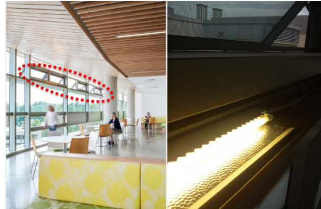
Figure 51. Environment Hall thermal corridor windows have lighting fixtures above that could be turned off during the day (Payette, n.d.)
