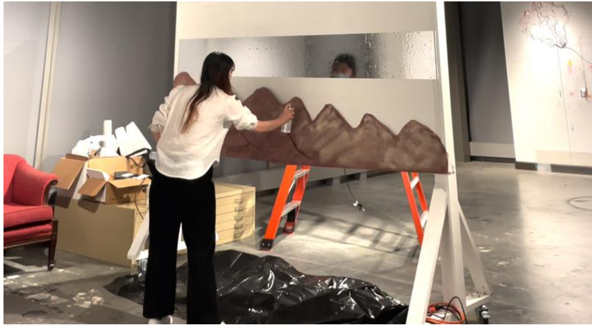
Figure 20: Rockery wall production process.
