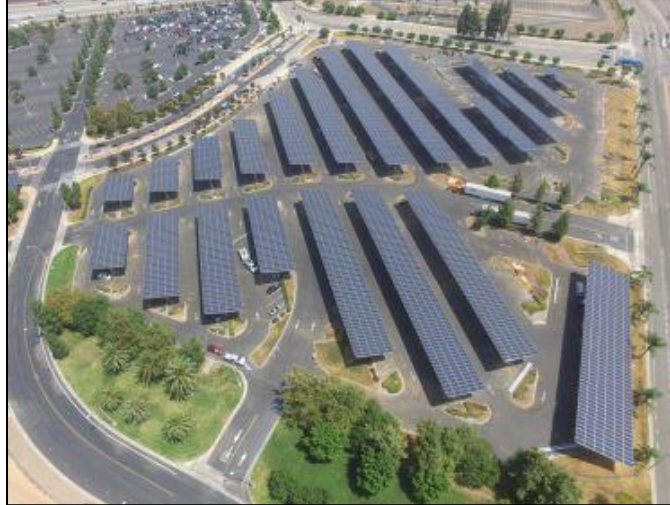
Figure 37. More than 9,600 solar panels are being installed in parking lots 30 and 32 at UC Riverside [83].
