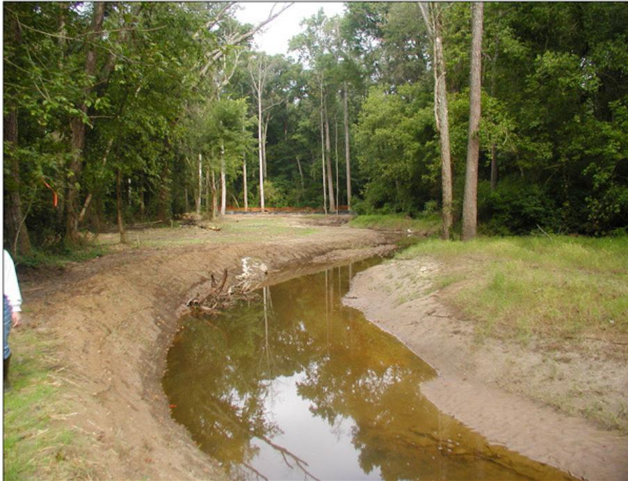
Figure 3: Post-restored Sandy Creek with restored sinuosity and floodplain in 2005. (Richardson 2007)
