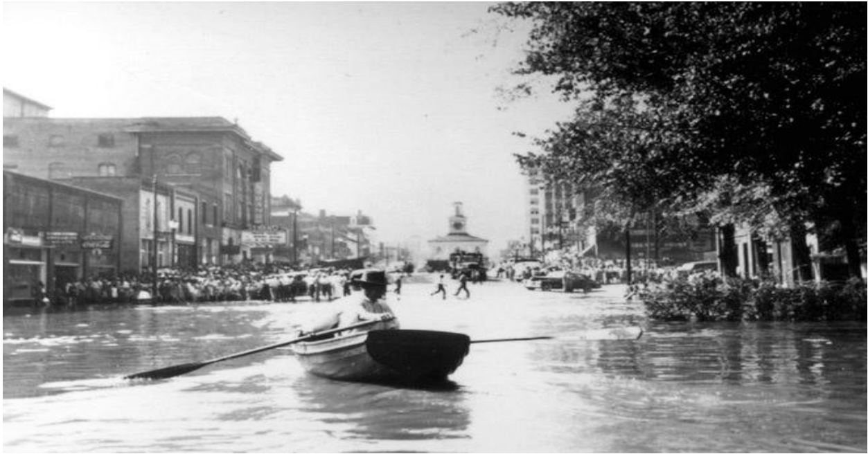
Downtown Fayetteville Flooded— Courtesy of The Fayetteville Observer, 2017
